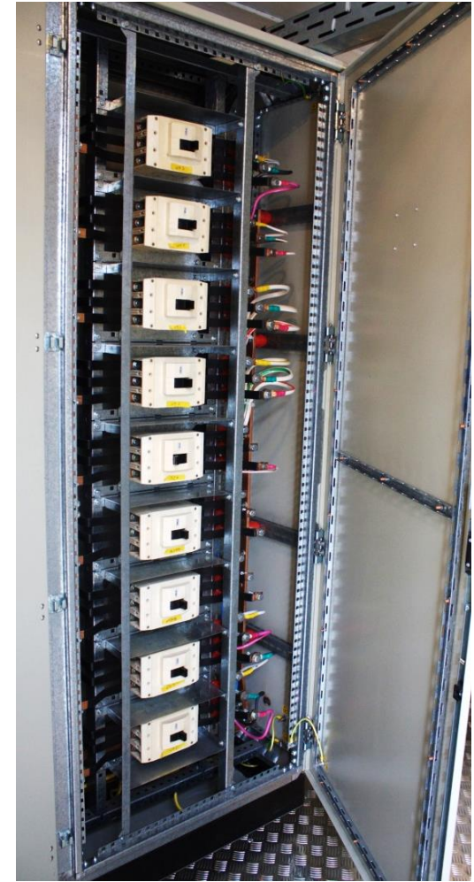
Distributing board and control cabinets
