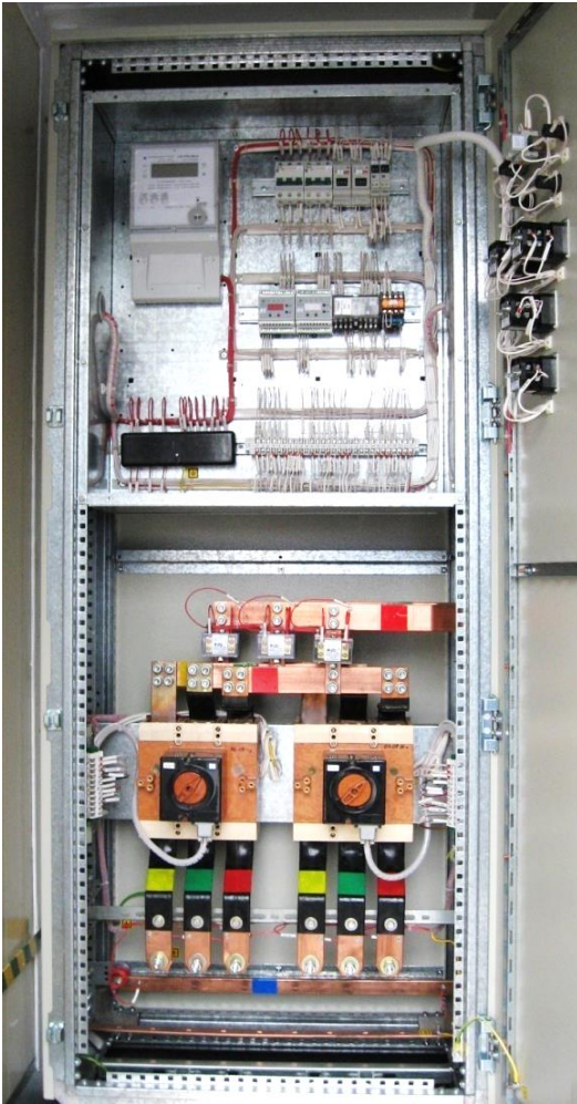
Incoming supply distribution assembly with the automatic transfer circuit-breaker in the block-box of the electric heating system
