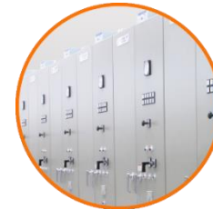
Electrical cabinets & automation systems
